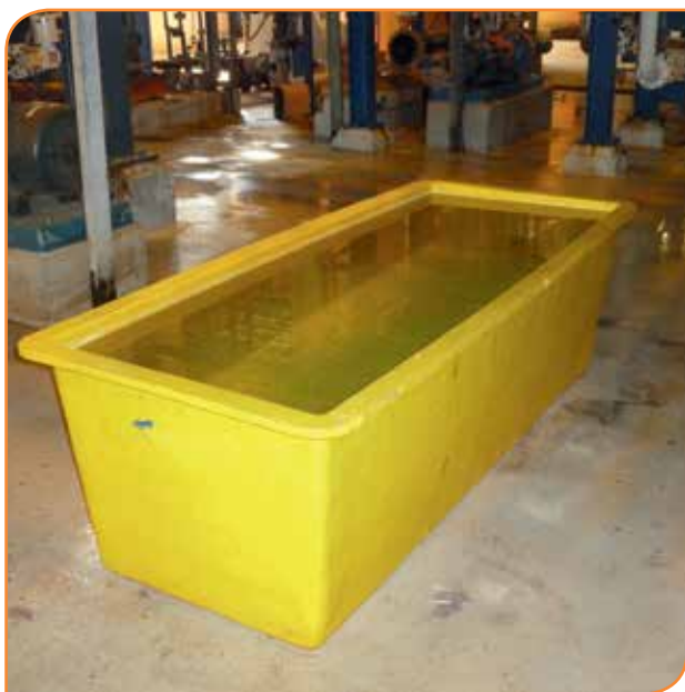
Jump tank installed at our Columbus, Mississippi facility
