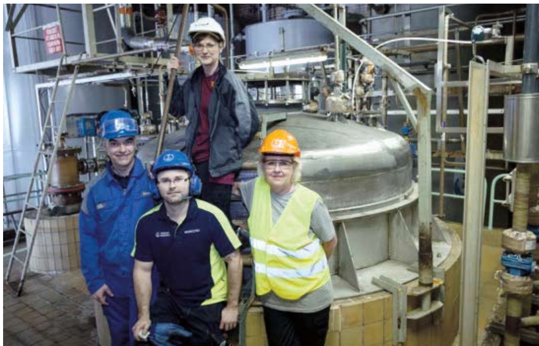
Iggesund's Hans Nilsson (left) and Morgan Arousell, process operator, at the retrofitted chlorine dioxide plant. Photo also includes Kimona Häggström and Helena Falgén with AkzoNobel.
